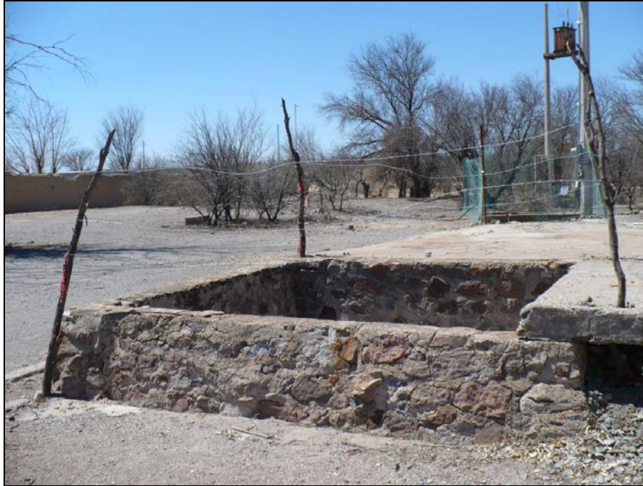
Figure 12-3: Water well at logging compound
