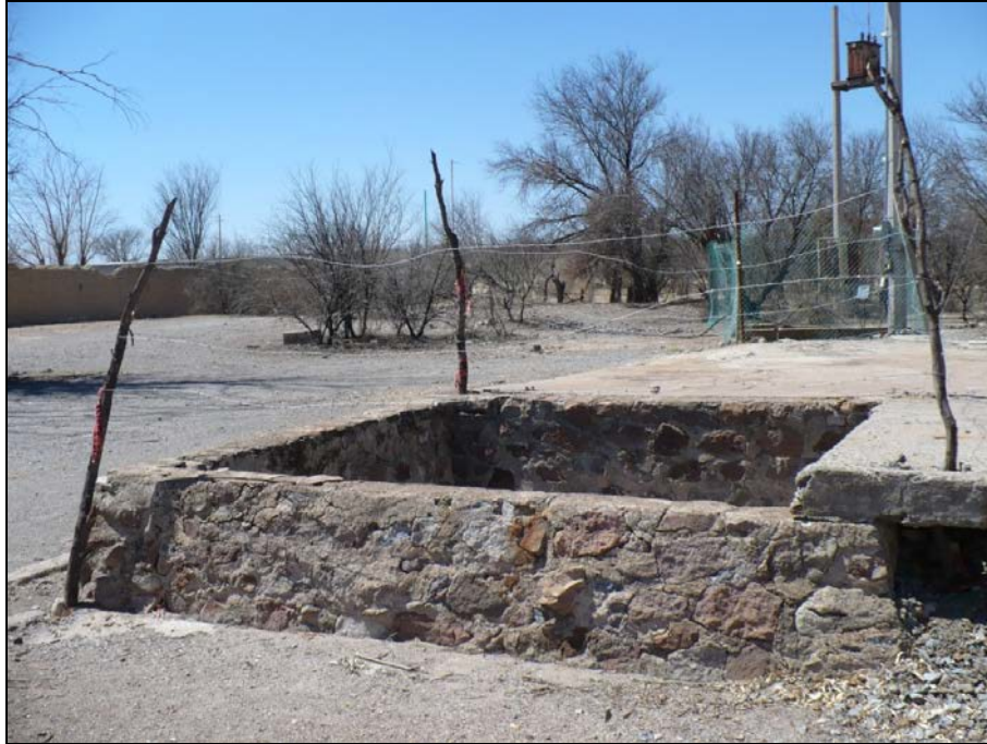
Figure 12-3: Water well at logging compound
