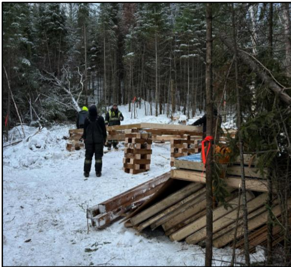
Figure 1: Rig Substructure Setup
