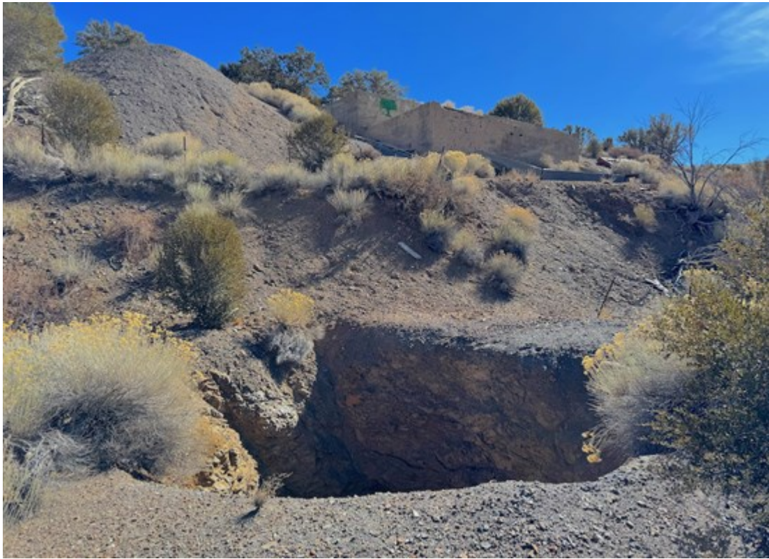
Figure 2: Looking northeast at the shaft - foreground, and dumps and concrete foundations behind.
