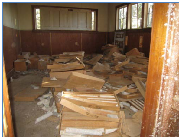
Destroyed core in building
