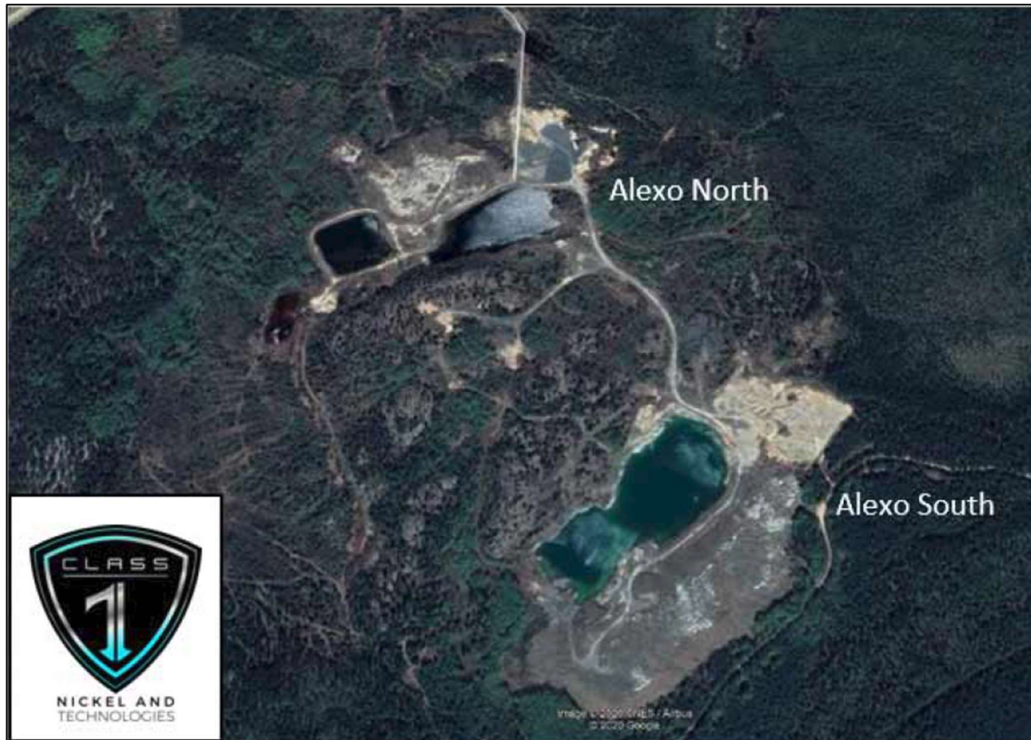
Figure 5-3. Google Earth image showing the location of historical infrastructure at the Alexo North and Alexo South mine sites (Donaghy and Puritch, 2020).
