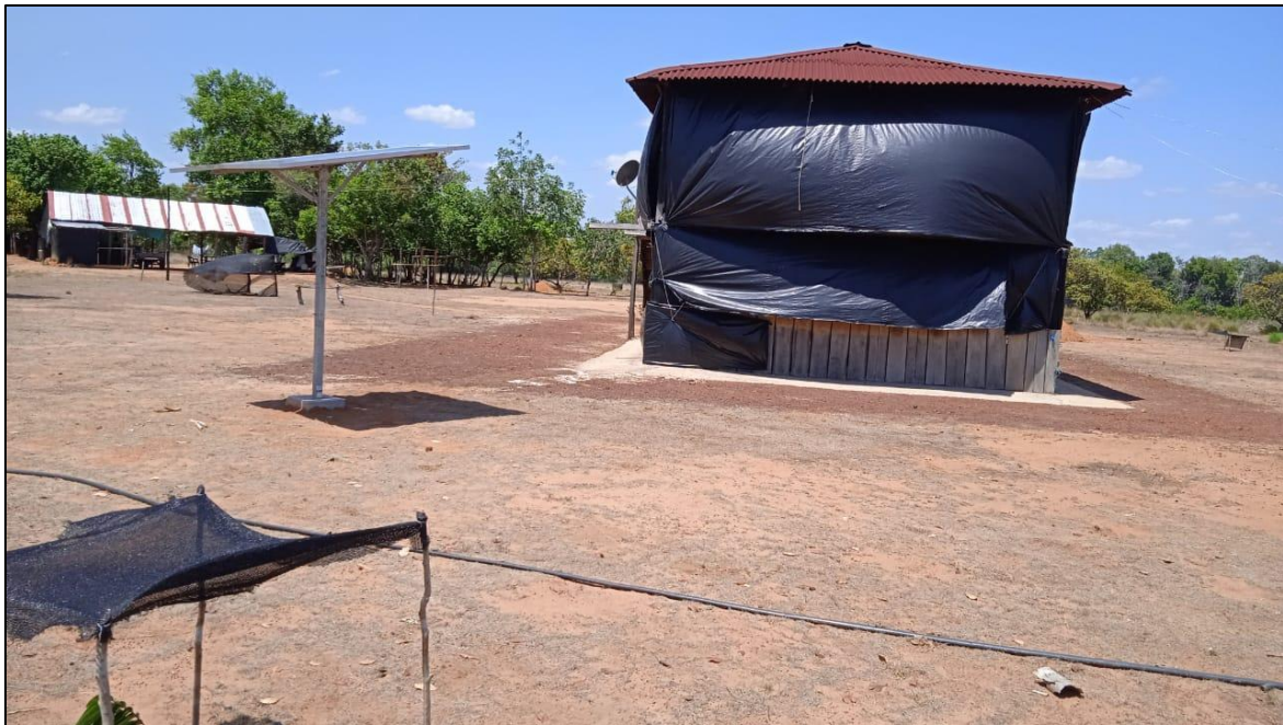
Figure 6. Minastyc camp infrastructure, solar panels, lodging and kitchen.
