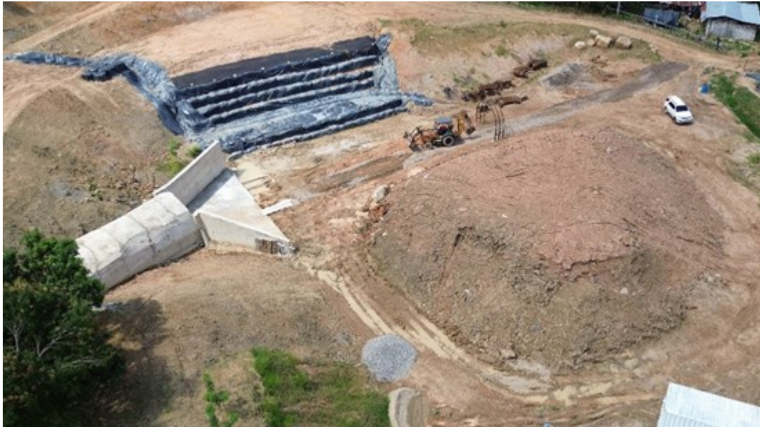
Figure 1. Works plaza and completed portal
