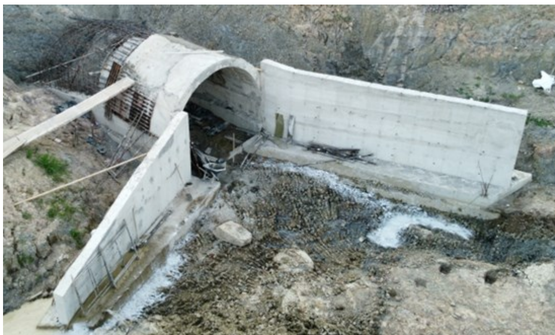
Figure 2 - Portal Construction Progress as of Jan 23, 2024
