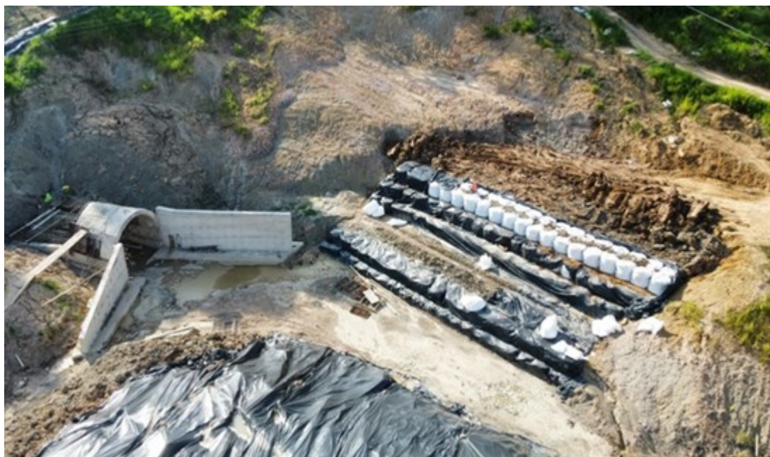
Figure 1 - Portal Construction Progress as of Jan 23, 2024
