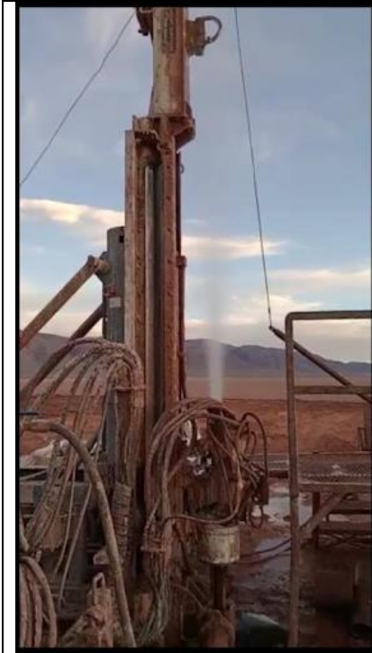
Fig 1. Dec, 2022 Drilling at Pocitos 1
