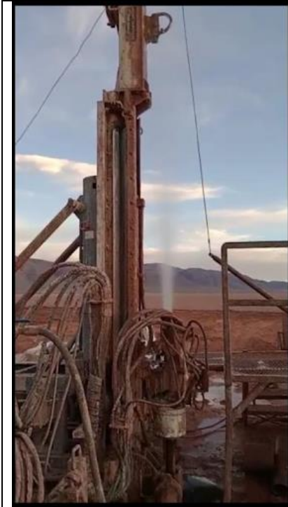
Fig 1. Dec, 2022 Drilling at Pocitos 1
