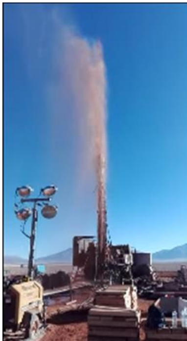
Fig 3. 2018 Drilling at Pocitos 1
