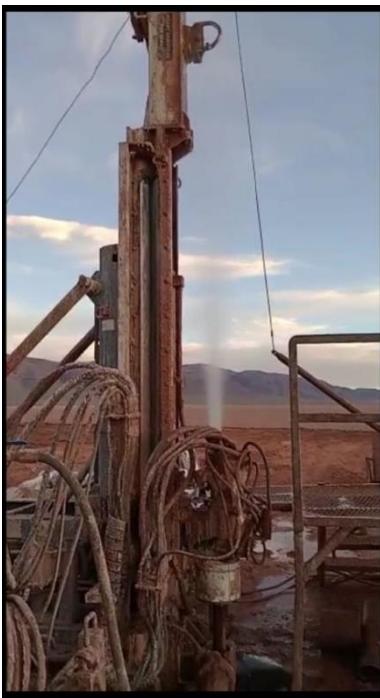
Fig 2. Dec, 2022 Drilling at Pocitos 1
