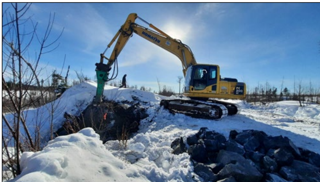
FIGURE 9.6 PHOTOGRAPH SHOWING EXCAVATION OF THE BULK SAMPLE
