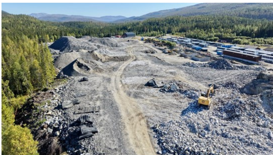
Norway Site 110MW Expansion Under Construction
